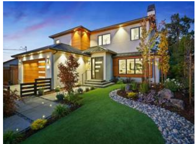
Leaver Construction 3218 Adelaide Way
