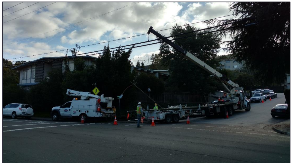
Pictured left and above - old pole and removal of pole
