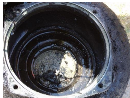
Wear ring and Impeller maintenance check
