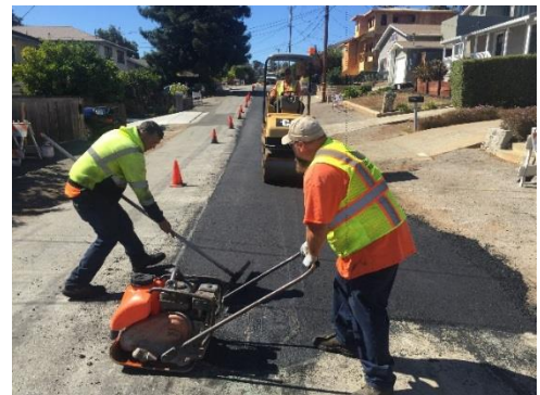
Monroe Avenue pavement repairs
