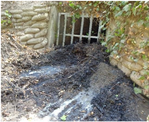
Water Dog Lake lower gate inlet-Before cleaning
