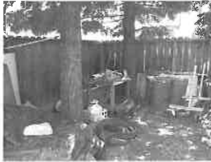
A close-up view of equipment, tools, and rubble stored under the canopy driplines of trees #1, 2, 3. All of this material will need to be removed prior to setting up the chain link root protection zone fence perimeter, wood chip mulch, and temporary irrigation.
