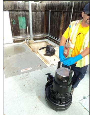
to the manufacturer's repair facility in Fairfield for repairs. This week Public Works received the rebuilt pump, and has since installed and tested the pump for proper operations. The pump station is now running at normal capacity.
