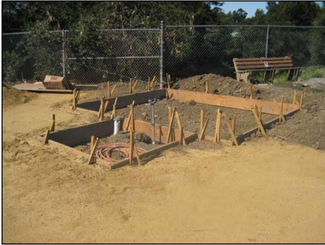
Construction continues on the renovations to the Cipriani Dog Park. The contractor is finishing the grading and the shade structure and doggy drinking fountain area are being built. Construction is proceeding on schedule
